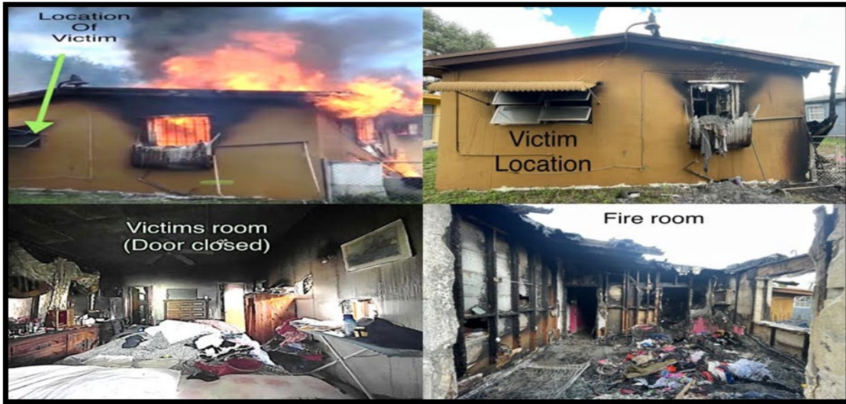
(FIGURE 2) THESE PHOTOGRAPHS ARE OF THE BATT 5 GRAB MENTIONED ABOVE. THEY SHOWCASE THE IMPRESSIVE CAPACITY OF A SIMPLE RESIDENTIAL INTERIOR DOOR TO EFFICIENTLY WITHSTAND SMOKE AND FIRE. BY MAINTAINING DISCIPLINE AND TAKING ADVANTAGE OF THIS POTENTIAL, WE EMPOWER OURSELVES TO REACH OUR HIGHEST LEVEL OF PERFORMANCE, AS R202 DID ON THIS FIRE WHICH RESULTED IN A SAVED LIFE.
